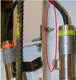
Figure 8 - Web-flange junction failure in column (1).
